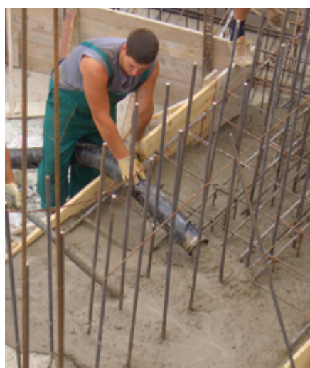
The P 718 conveys fine concrete up to a grain size of 32 mm, among other things.
